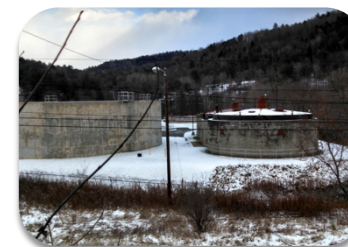
Major infrastructure failure
