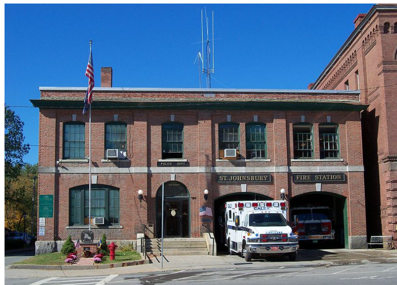
St. Johnsbury's historic downtown fire station has major limitations for fighting fires and assisting neighboring towns.
